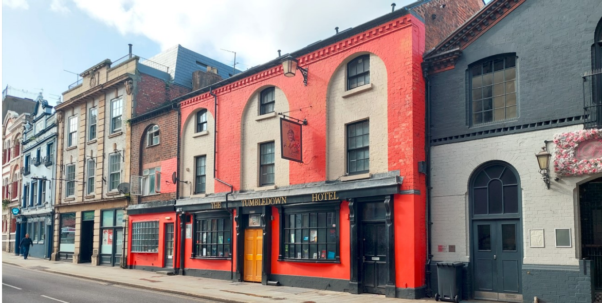
- Front view of the premises from Castle Foregate –
